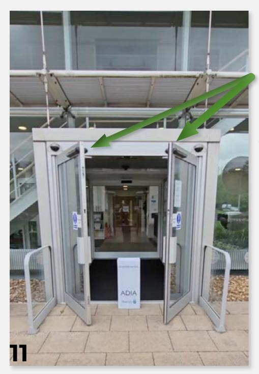
On door safety sensors, reducing the risk of impact and crushing within the sweep area of the door.
