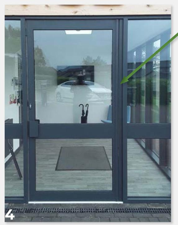
The frame of the door is curved at the pivot point to eliminate any trapping risk.
