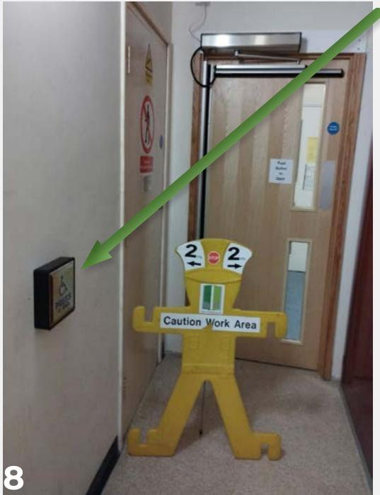
Push pads, installed at 1000mm for wheelchair and persons requiring assistance.
