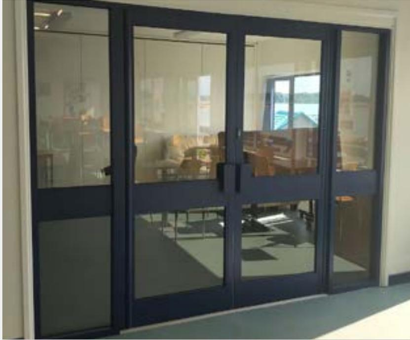
A pair of aluminium doors with a side light frame
