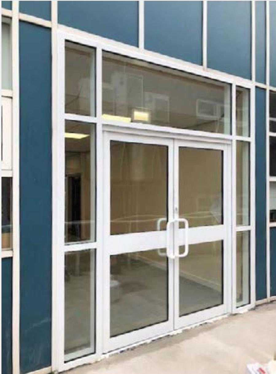
A pair of aluminium doors with a side and fanlight frame
